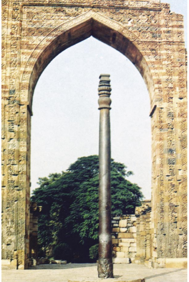
The 1,600-year-old Delhi Iron Pillar exhibits very good corrosion resistance despite its age. Photo courtesy of R. Balasubramaniam, IIT Kanpur.
