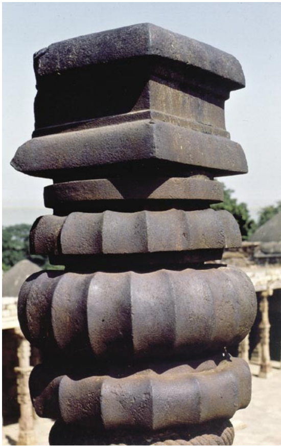
These photos show the upper and lower sections of the decorative bell capital atop the Delhi Iron Pillar. The different components were shrunk-fit around a hollow cylinder. Photos courtesy of R. Balasubramaniam, IIT Kanpur.
