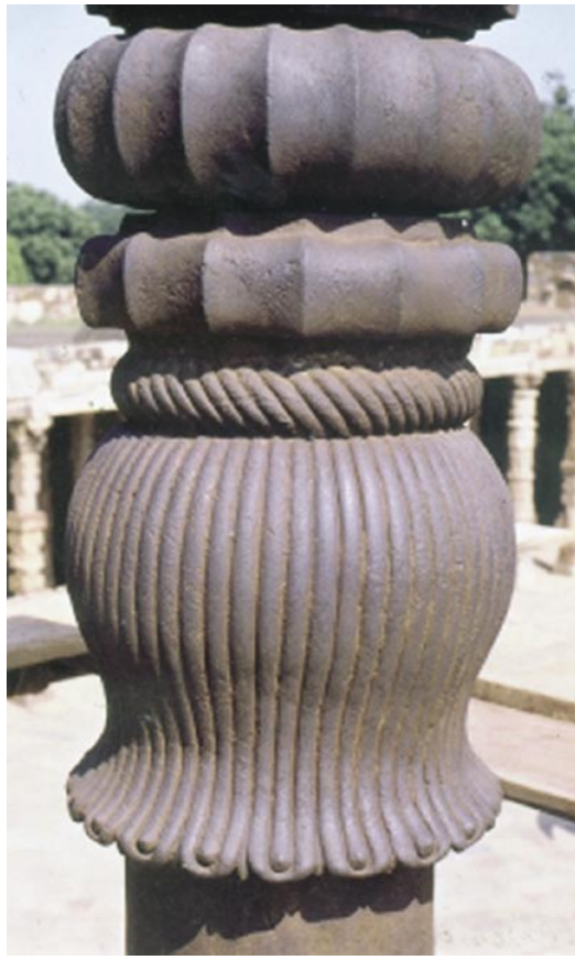
These photos show the upper and lower sections of the decorative bell capital atop the Delhi Iron Pillar. The different components were shrunk-fit around a hollow cylinder. Photos courtesy of R. Balasubramaniam, IIT Kanpur.
